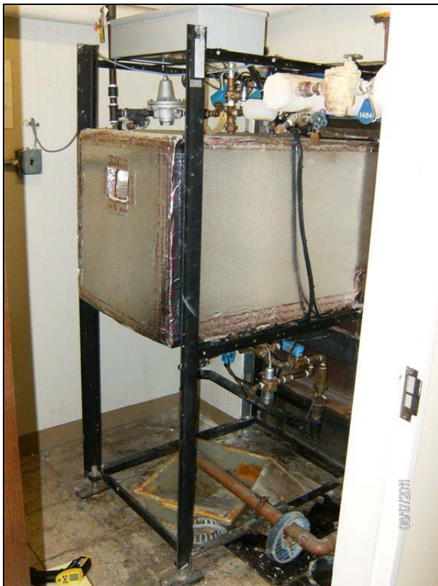
Figure 7 Autoclave in Fordham hall whose drain was modified to conserve water.
